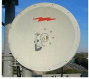
Dishes 3 feet in diameter or greater can have an input of up to 1 Watt with no areas exceeding FCC General Public exposure limits. The more common 1 foot dish can have input powers up to 100 mW and remain below limits. Square antennas can have slightly higher power for their size (width) and remain below limits.
